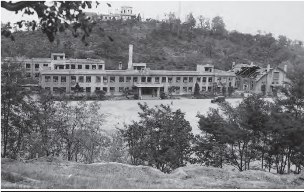
FIGURE 7-2. The Korean civilian hospital in Incheon, Korea, was operated by the 1st MASH and had little or no supplies initially (3 October 1950). Fixed facilities were much better than canvas tents and were utilized whenever possible. Photograph courtesy of the AMEDD Center of History and Heritage, Army Nurse Corps Photo Collection, Korean War, Box 25, Item #B4-03-02(1).
