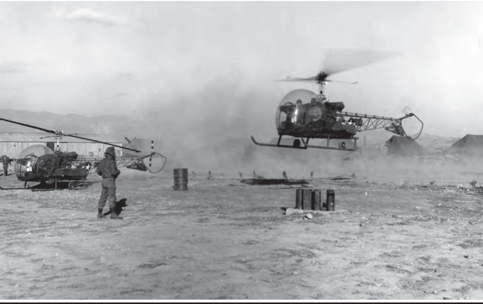
FIGURE 7-1. Captain Joseph W Hely of St Louis, Missouri, 2nd Helicopter Detachment, 2nd Logistical Command, lands a Bell H-13 at his detachment headquarters following an evacuation from the front (31 December 1950). Note the litters covering patients like a “casket,” and skids replacing the wheeled landing gear. Photograph courtesy of the AMEDD Center of History and Heritage, Army Nurse Corps Photo Collection, Korean War, Box 25, Item #B4-O4-02(1).
