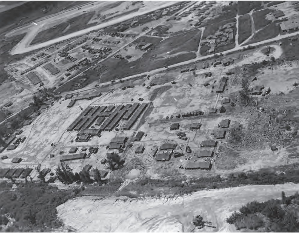
FIGURE 7-4. Aerial view of the 8076th MASH in Chounchon, Korea (29 July 1951). Note the Basic “U” used to build the tented hospital. It was here that the core functions were established—preoperative, postoperative, and surgical wards. Photograph courtesy of the AMEDD Center of History and Heritage, Thomas N Page Collection, Box 4, Image #8A/854-9/FEC-51.
