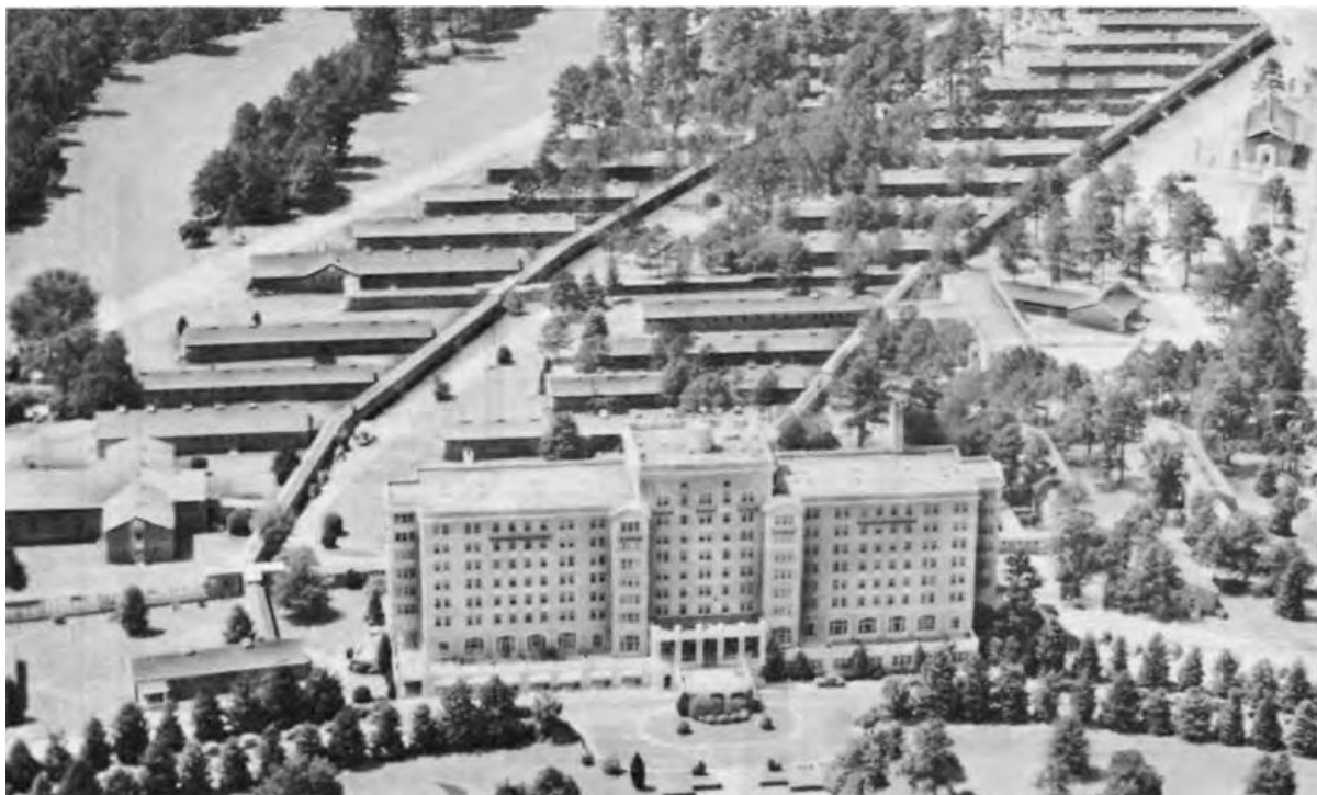
OLIVER GENERAL HOSPITAL converted from the Forest Hills Hotel.
